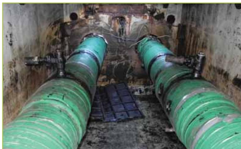
**Figure 6. Photograph of underground high-pressure, fluid-filled feeder cable joints.**
